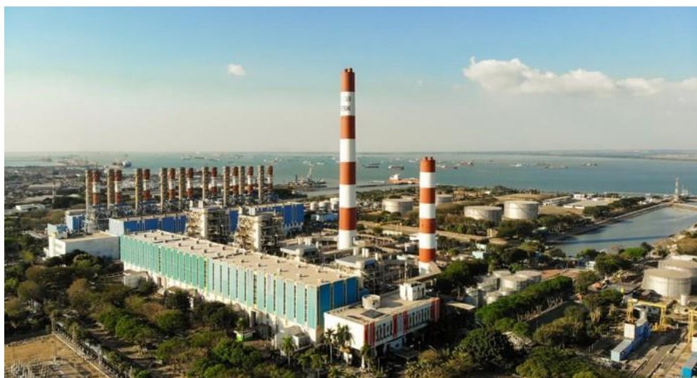
Figure 1. PLTU Suralaya Power Plant
